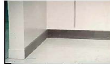
Corner of a room
